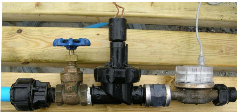
Figure 3 - A typical commercial greenhouse set-up with an isolation tap, a 24 V electronically-controlled water valve and a water flow meter. See Appendix for details.
